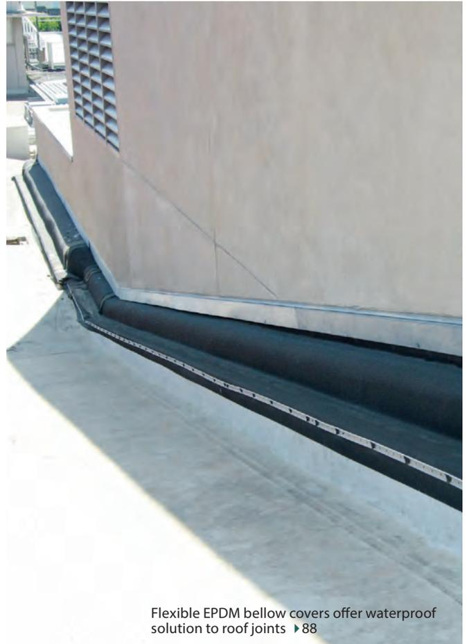
Flexible EPDM bellows covers offer waterproof solution to roof joints ▶ 88
