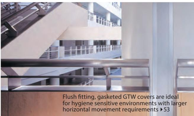
Flush fitting, gasketed GTW covers are ideal for hygiene sensitive environments with larger horizontal movement requirements ▶ 53
